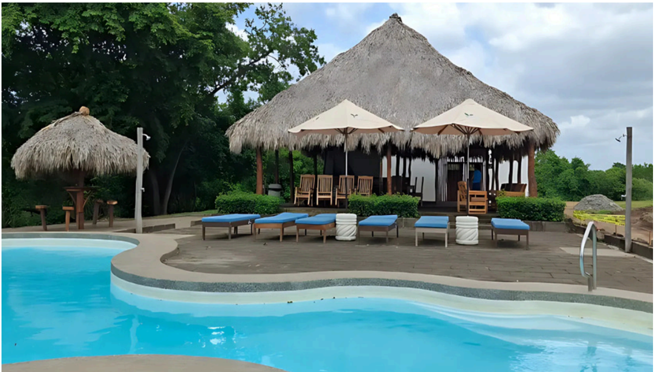
Photos of the EVA community and completed amenities at Gran Pacifica in Nicaragua as of December 2024.
