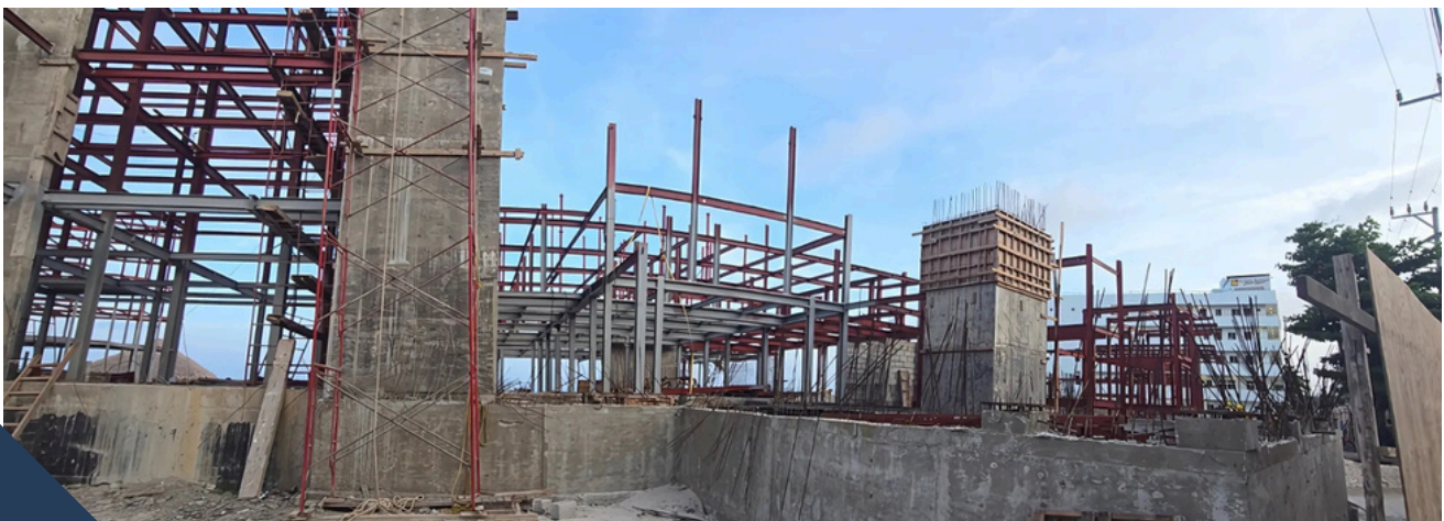
Construction photos of the Marriott® Residences in Belize as of November 2024.
