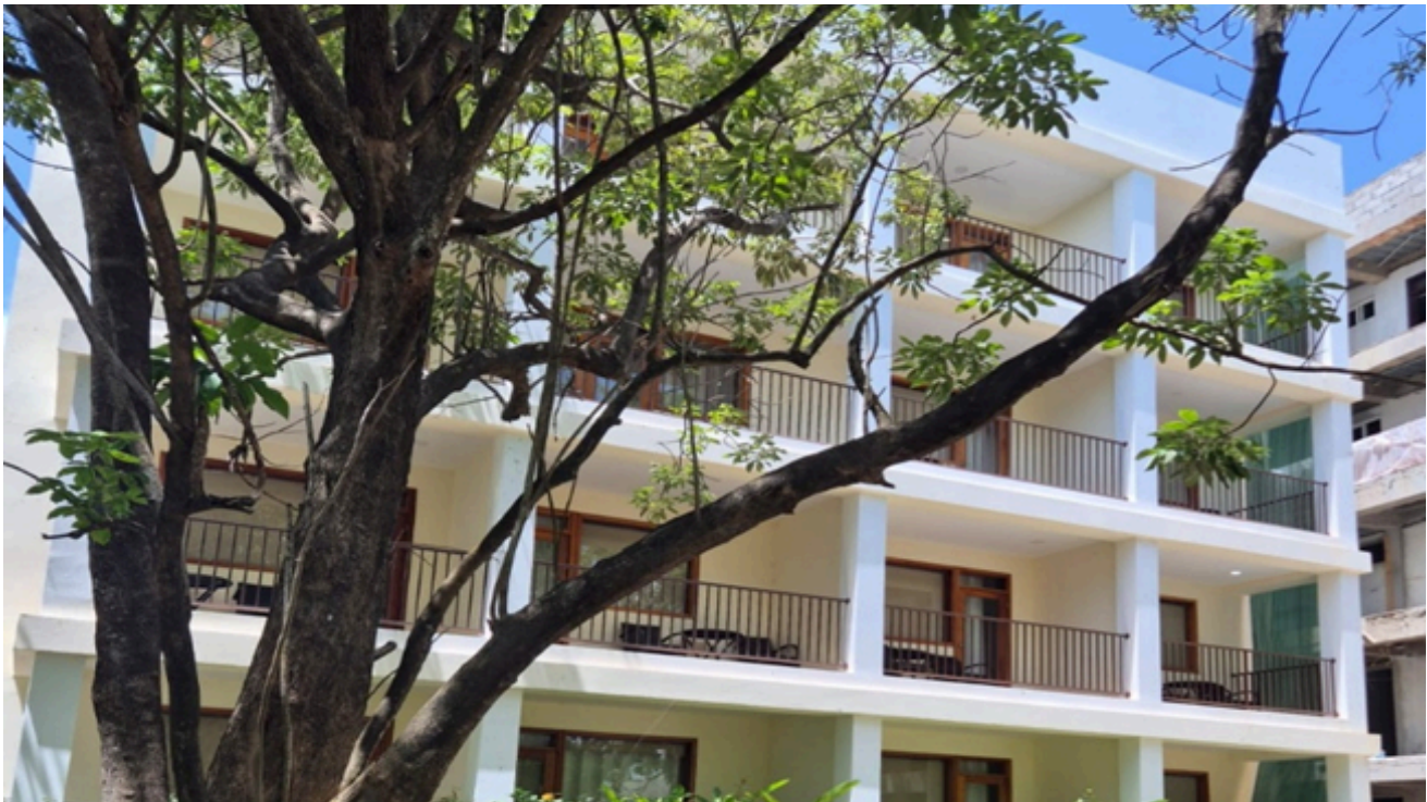
Completed Fleet building at Grand Baymen Gardens as of 2024.
